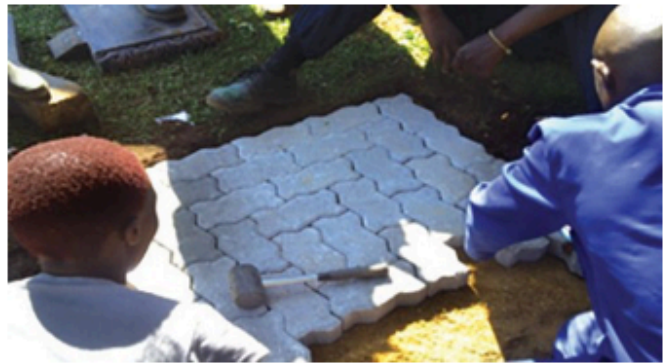
Learner being taught how to lay paving
