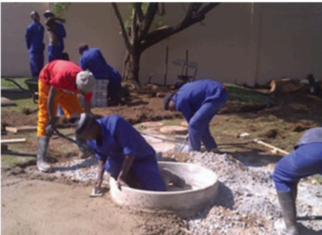
Learners installing concrete paving and water feature
