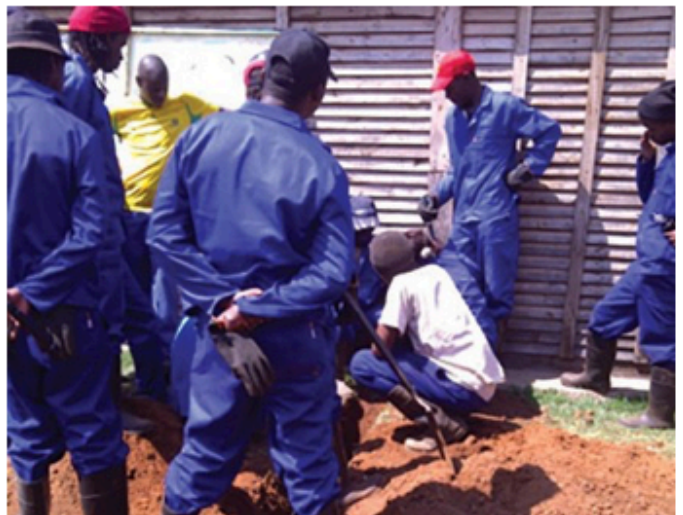
Learners installing irrigation equipment
